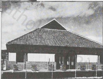
ST. MARGARET CLITHEROW, WHINMOOR, LEEDS under construction. ▼
